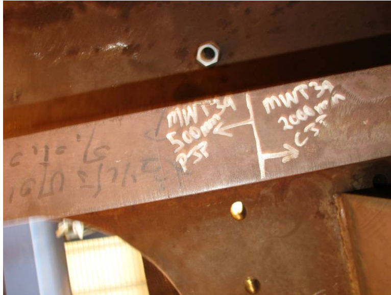
Photograph 5: View of the weld status markings noted on the ABF mock-up.
