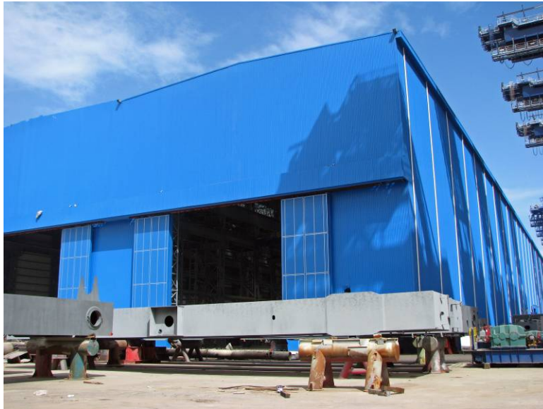
Photograph 1: Overall view of the exterior of the new Tower Fabrication facility.
