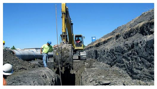
The Altamont Pipeline project consists of approximately 12 miles of 42-inch to 48-inch diameter transmission pipeline that will connect the Altamont Water Treatment Plant to the Zone 7 distribution system.
